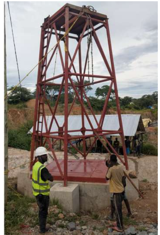
Headframe installation
